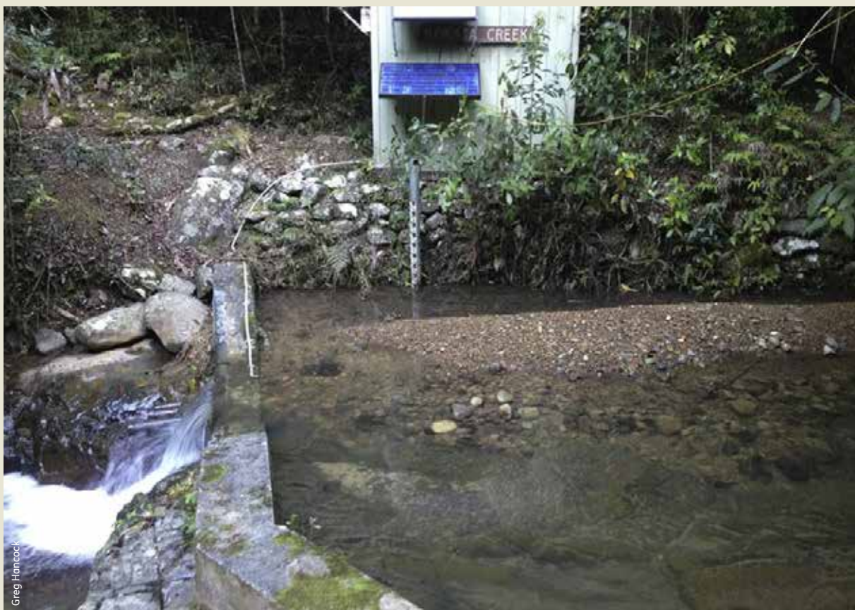
Stream flow and sediment monitoring weir, Karuah catchment research, NSW.
