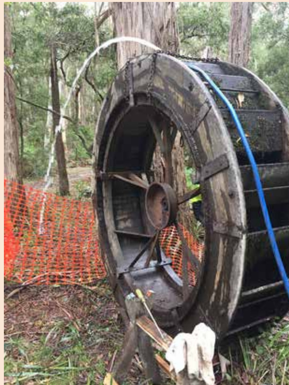
Figure 6.30: Historic water wheel under repair, Lowden Forest Park, New South Wales
